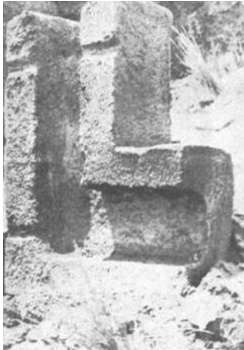
The angled section of a water conduit from Tiahuanaco Protective tubes for energy cables?
